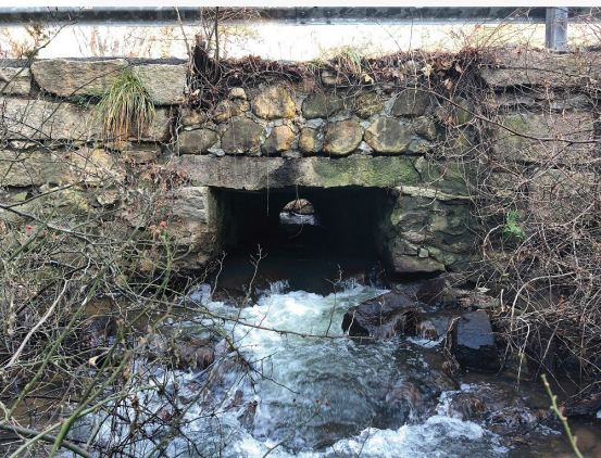
Town of Mashpee Santuit River Culvert
