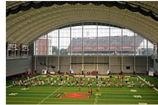
Cole Field House Performance Center Interior facing north, 2017
